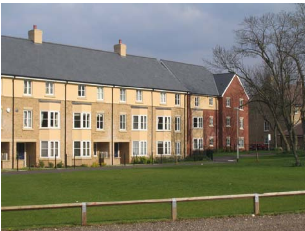
Large scale mixed use infill development, Papworth Everard. Buildings include townhouses and flats around a new public open green space and a new public library with retail development.
